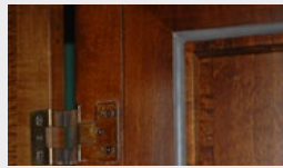
Rubber gasket allows for expansion & contraction
